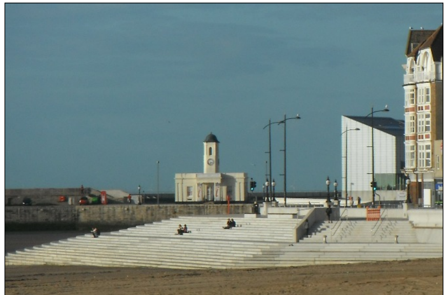
The Harbour Steps flood prevention works
