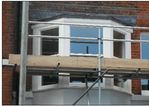
Close-up of one of the replacement windows
