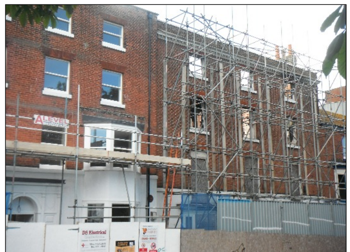
This photo shows Nos 47-48 Hawley Square on the left and Nos 49-50 Hawley Square on the right (All the photos in this page were taken on 19th August 2015)
